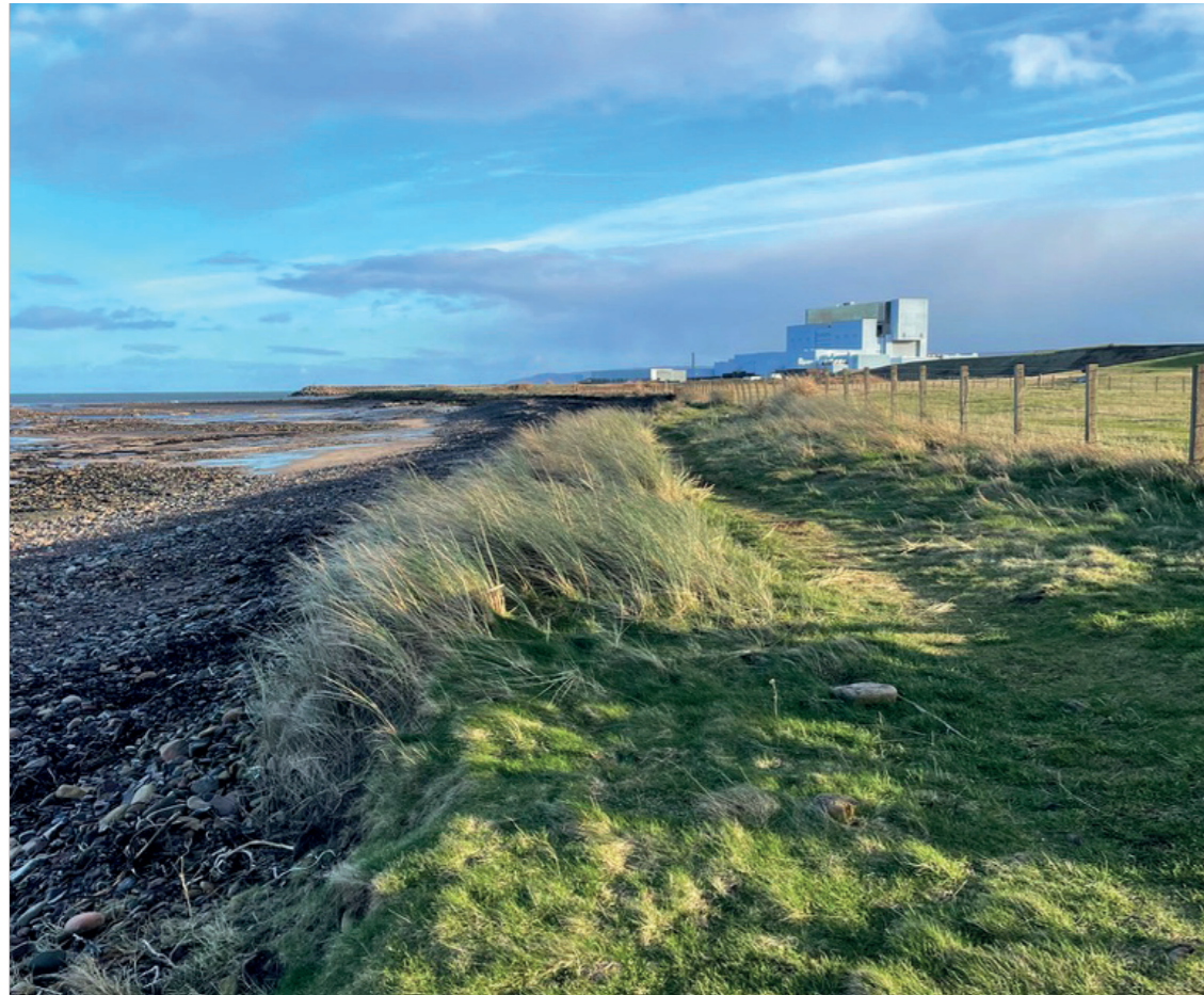
4 - John Muir Way, southeast, towards proposed landfall location and Torness Power Station.
