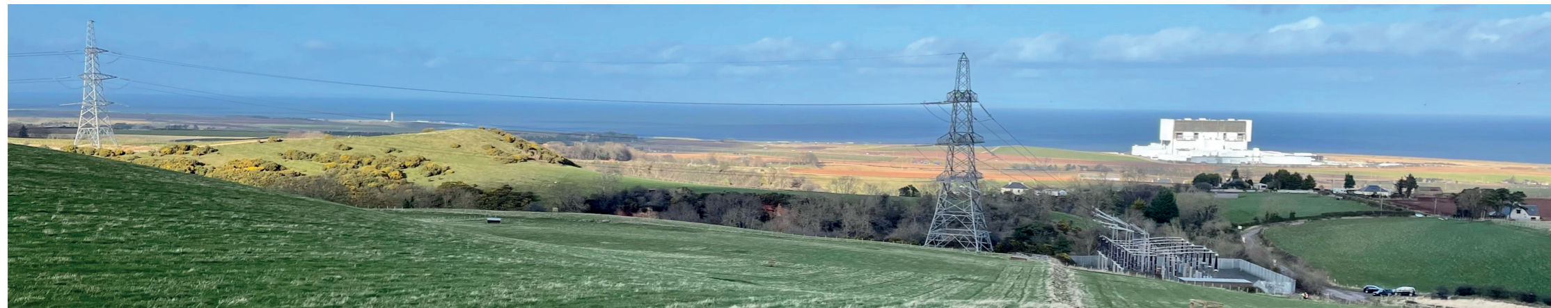
14 - Southern most extent of onshore cable corridor approaching the proposed Branxton Grid substation, south of the Braidwood Burn and existing OHL and Innerwick substation.
