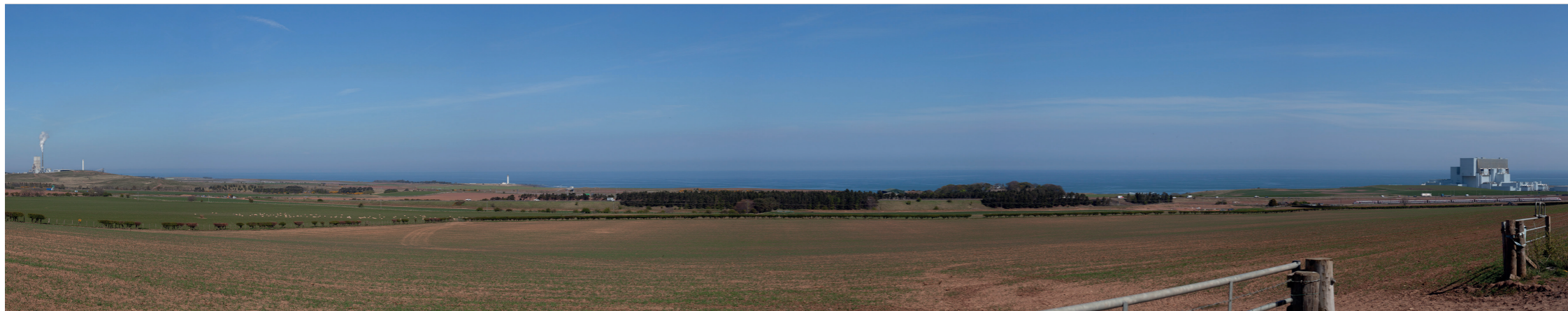
8 - Existing influences on the East Lothian coast include Dunbar Cement Plant, Dunbar Energy Recovery Facility and Torness Power Station. The ECML also passes the northern site boundary.
