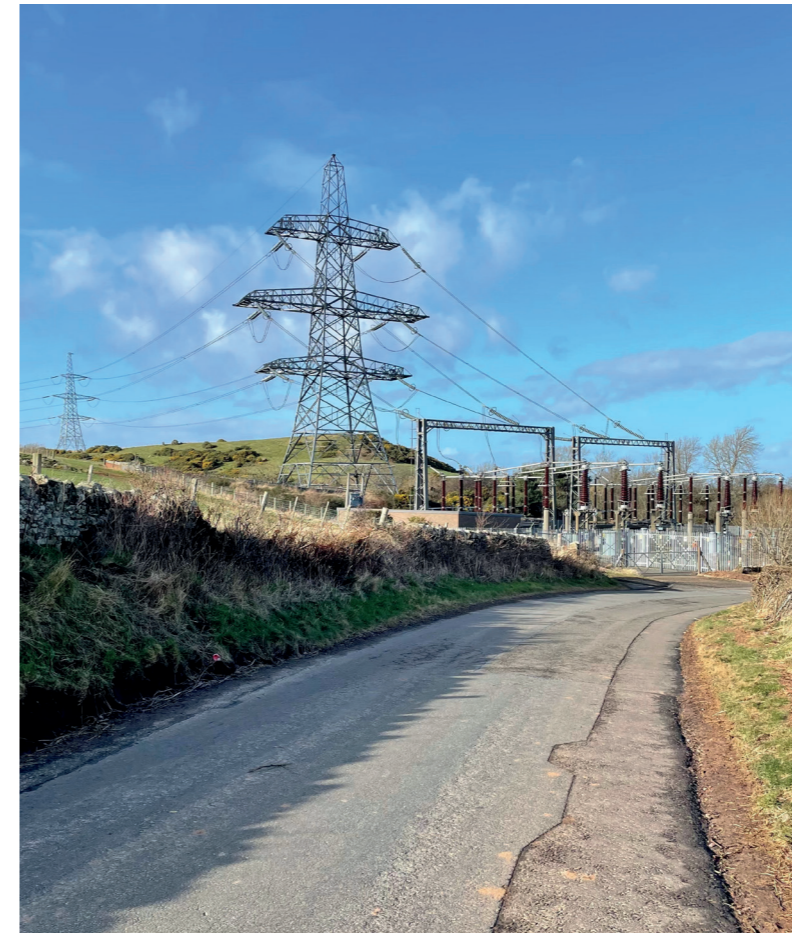
13 - Existing Innerwick electricity substation.
