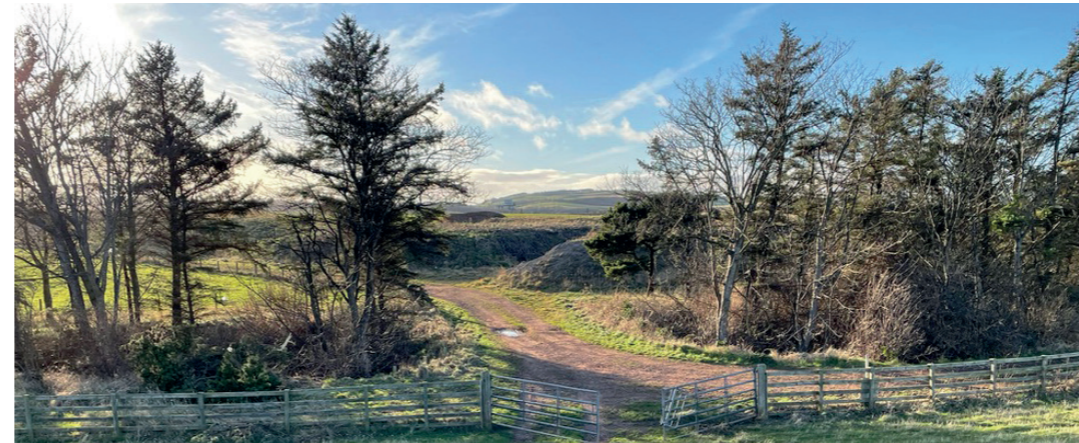
5 - Onshore cable corridor includes proposals to widen existing culvert to Dry Burn.
