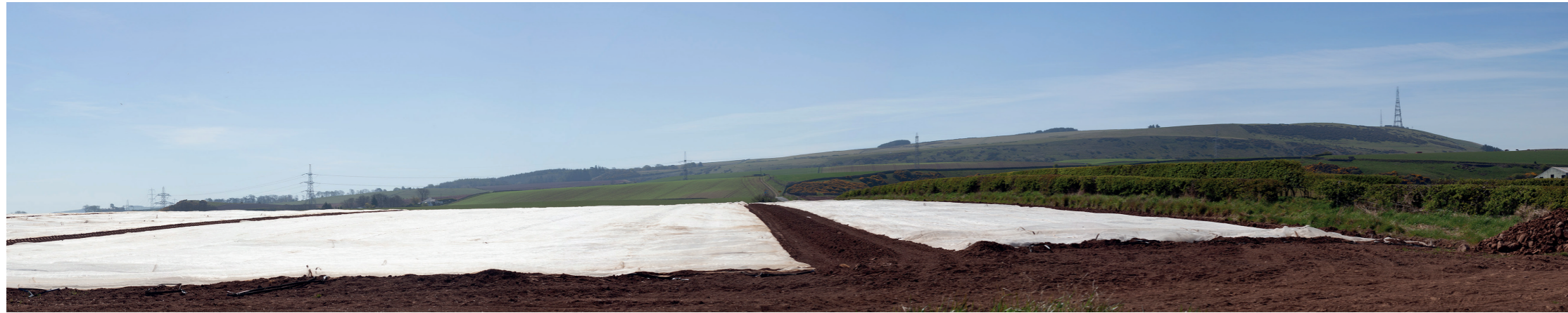
10 - Onshore substation to Branxton Substation cable corridor, looking south. Foothills form backdrop of inland views from the coast with existing OHL and Blackcastle Hill radio tower visible.
