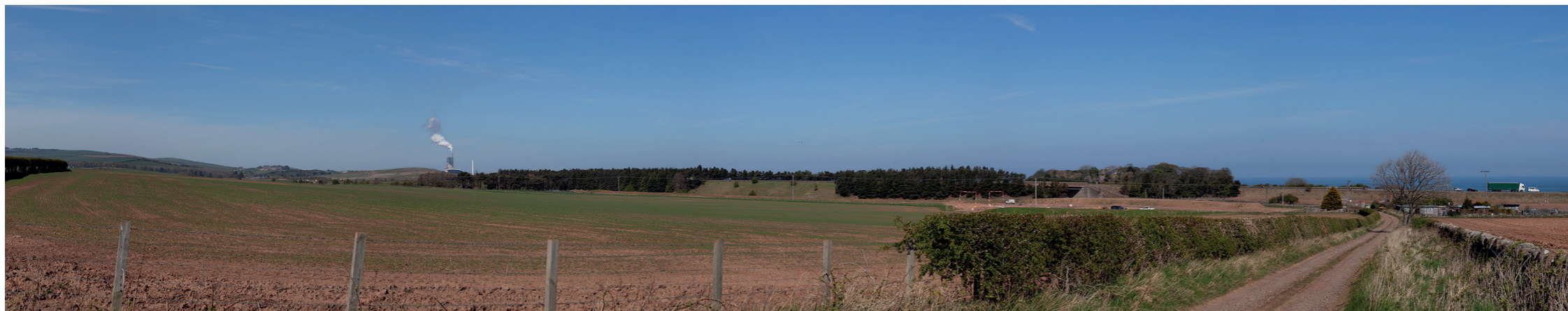
9 - Proposed onshore electricity transmission buildings (indicative) site, viewed from eastern farm access track. Shelter belt planting following carriageway of A1 contains visibility to onshore cable route, to north.
